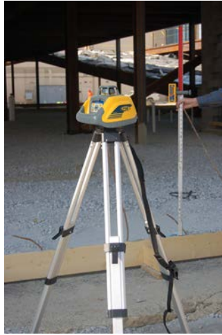
Exterior application setting forms
