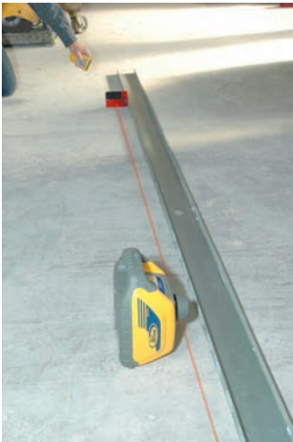
Vertical alignment application
